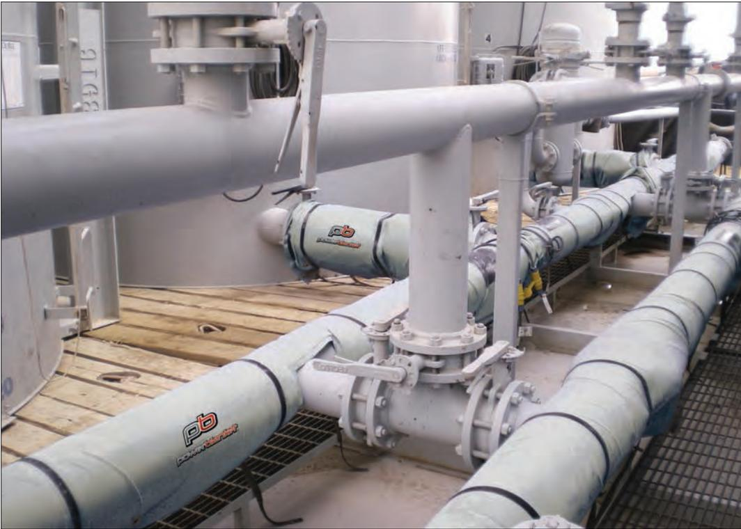
On-site Pipe & Manifold Heating System
