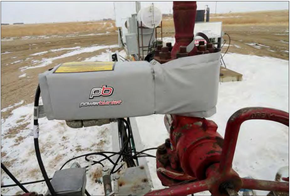
On-site Valve & Instrumentation Heater
